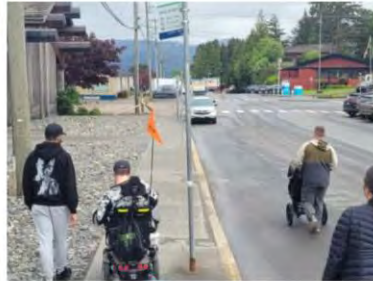
Narrow and obstructed sidewalk
