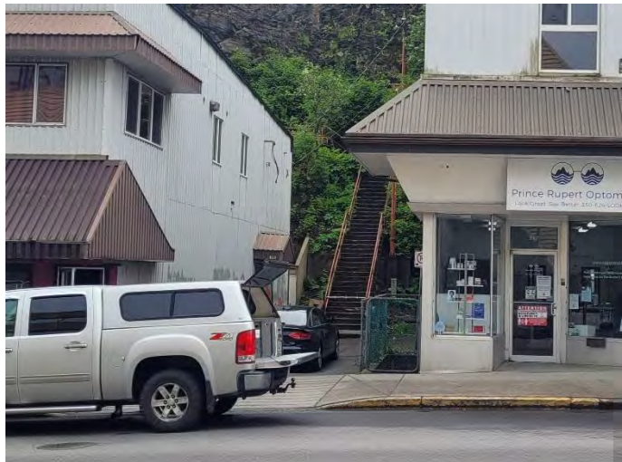
Closed staircase on 3 rd Avenue West
