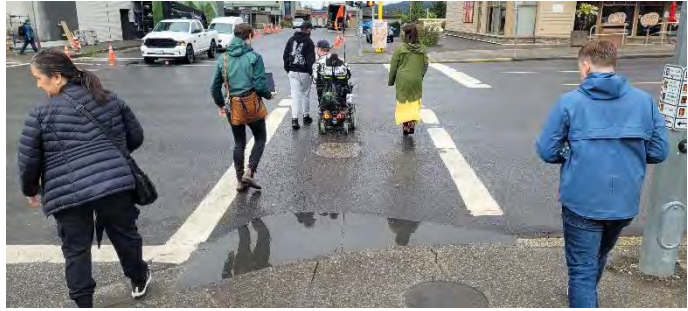
An intersection with poor drainage
