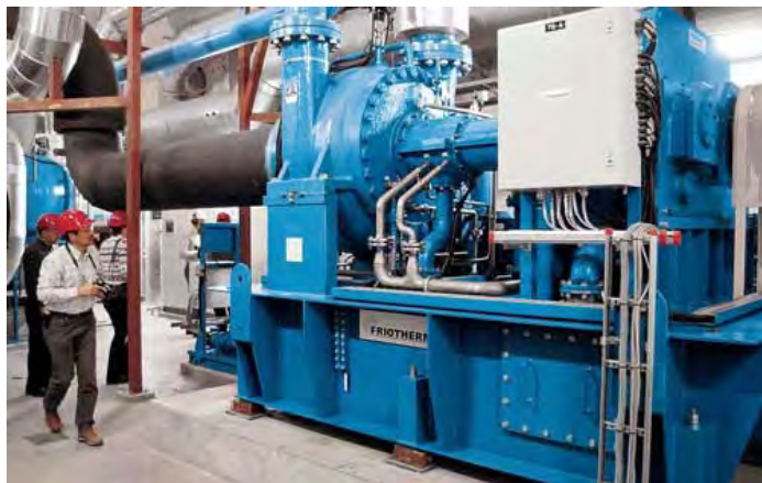
Figure 3-2 Installation of Heat Pump (18.4 MW) Equipped With Shell and Tube Heat Exchangers for Heat Recovery from Raw Wastewater
