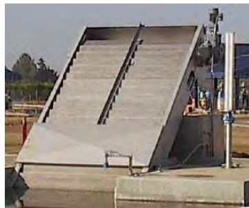
Photo of Escalator Fine Screen courtesy of John Meunier, Inc.
