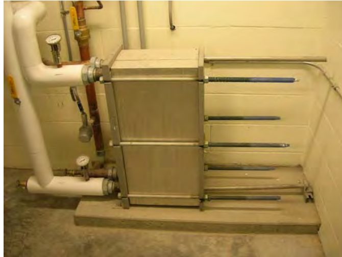
Figure 3-1 Example of Pumped Plate and Frame Heat Exchanger Installed in a Water Treatment Facility that Uses Lake Water for Heating and Cooling
