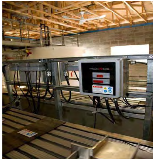
Figure 7-2 Typical UV Lamp Bank
