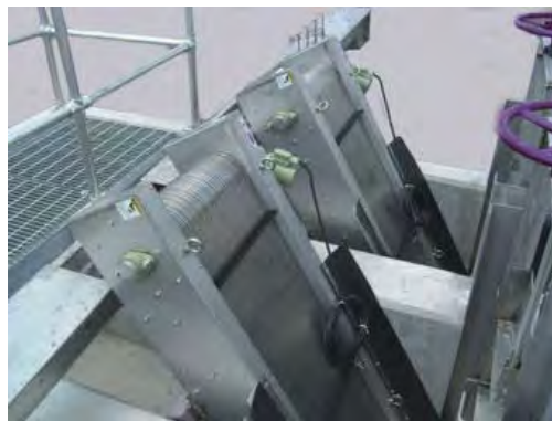
Figure 3-2 Example of Fine Screens
